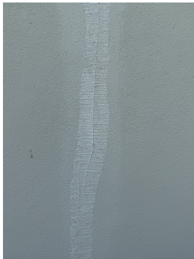
Apply the patch. Work the selected elastomeric material into the prepared crack with a putty knife.
