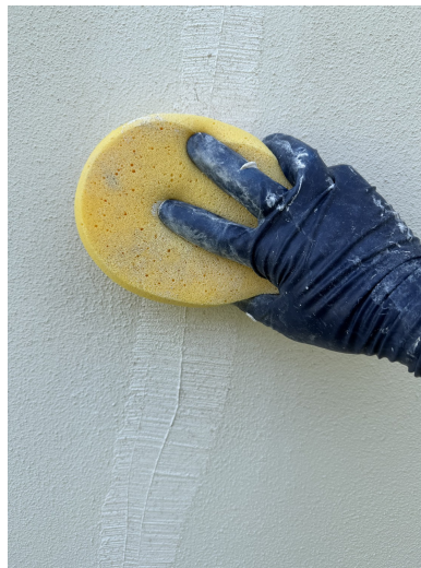
Blend with the sponge. Tap the workable material to remove excess and match the adjacent texture, including the repair edges.
