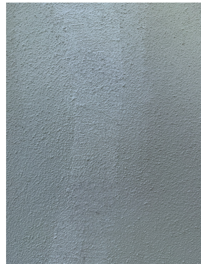
Check the texture. Inspect the transition into the existing stucco, then allow the required cure before priming and painting.
