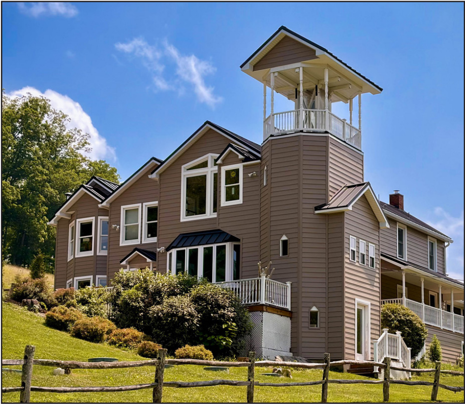
The renewed exterior, with its new roof, siding, and windows.
